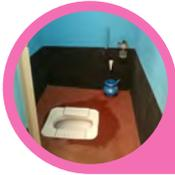
**Pour-flush latrine:** Pour-flush latrines provide an improved option in terms of use, maintenance and construction. They are a cross between a pit latrine and a septic tank or sewer. A small amount of water is used to flush excreta out of a collection pan, down a short pipe and into a pit. The simplest form of pour-flush latrine is the installation of a pan with a water-seal in the defecating hole over a pit.
