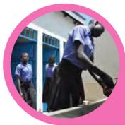
**Wash basins (group or individual):** Wash basins, connected to a piped water or gravity-flow system, are considered the best option as they provide sustained clean water for drinking and handwashing throughout the day.
