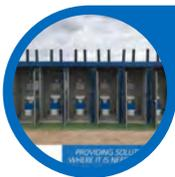
**Amalooloo toilets:** The **Amalooloo** is a unique sanitation system for both waterborne and dry (ventilated improved pit) structures. The scientific principle behind the technology is aerobic, natural composting of human excreta that is separated at source. The technology is only dependent on natural, environmental conditions resulting in ecologically friendly results. It also does not require water to function (but it is recommended for health and hygiene reasons).
