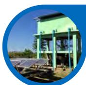
**Solar powered water systems:** A climate-resilient option which can make use of Lesotho's plentiful sunlight to pump water from deep in the ground - without expensive fuel and maintenance costs for the school. Storage containers are a central part of the system, providing extra water supply for periods of drought and can provide gravity-fed water supply to handwashing/drinking water tap stations (see Appendices, Fig.5 for more information).
