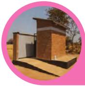
**A ramp with handrails or a smooth pathway leading to both sides of the toilet block:** This helps facilitate learners with motor disabilities to access the toilet block. A gradient of 1:15 or 1:20 for ramps is advised depending upon the availability of space. They should not be less than 1200mm wide (see Appendices Fig.13 for more details). Railings should also be provided for ramps where resources are available.
