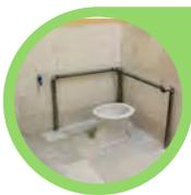
**Grab Rails:** Designed to improve learners' safety and help with mobility in and around the toilet cubicle. Must be secured and easy to grab hold of to maneuver.
